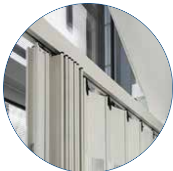
Guida superiore Top-hung track
